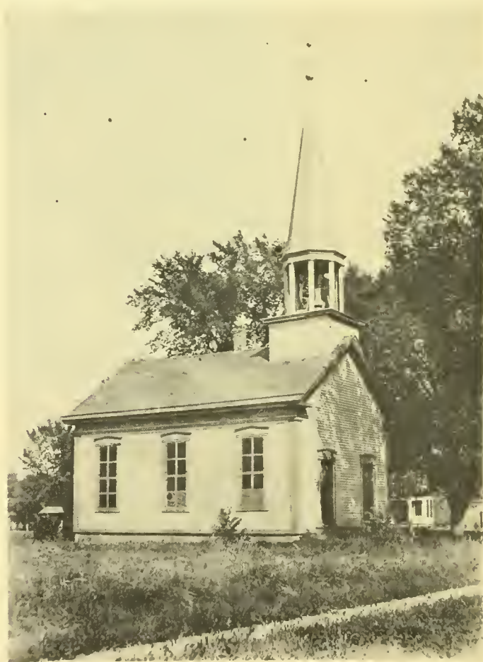
This picture of the Congregational Church was taken by Roy Francis McNabney about 1914. This church was built in 1856 by William Henry Luce, and he probably drew the plan. It is purely New England in design, the lines are good and the proportions harmonious. When it was painted white with green blinds, and the weather vane and the balls above and below it were covered with gold leaf, it looked as tho it might have been picked up from the hills of Maine or Vermont and transplanted out to the banks of the Mississippi. This was as it should be for the builder and most of the early members came from New England, and they wanted a church to remind them of the ones they attended when they were young.
