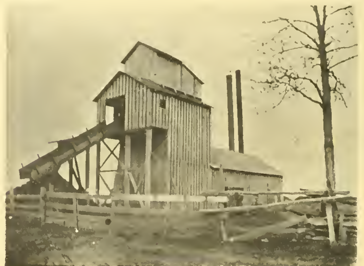
The Odendahl Shaft at Tinkerville
