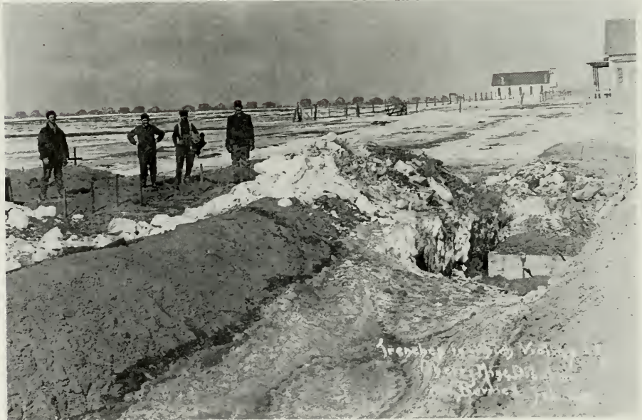
Huge trenches had to be dug to provide burial for the scores of victims that were laid to rest in the plot which was to become Cherry's Memorial Cemetery.
