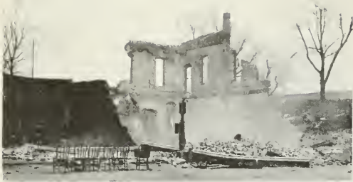
K. P. Lodge—Built 1906, Demolished 1929
